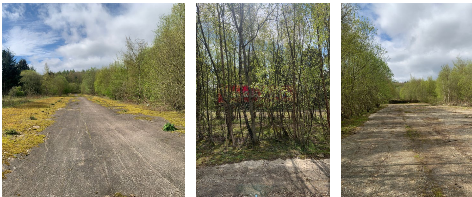
Existing site photo: historic concrete surface with self-seeded trees
